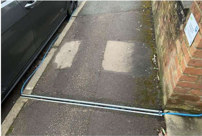
Figure 29: Charging Cable Gully (Leighton Buzzard Observer, 2022)
